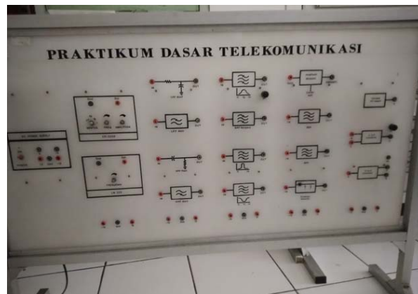
Figure-10 Basic Telecommunication Laboratory
