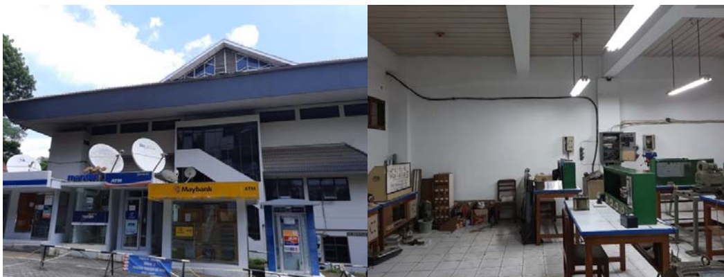
Figure-23 Locations for PV arrays and indoor system for SCU Microgrid Laboratory
