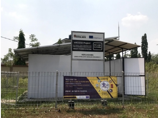
Figure 10. Atma Jaya University Photovoltaic Laboratory
