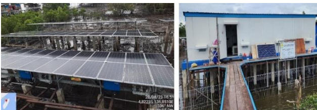
Fig. 11. 50 kWh Amamapare PV System
